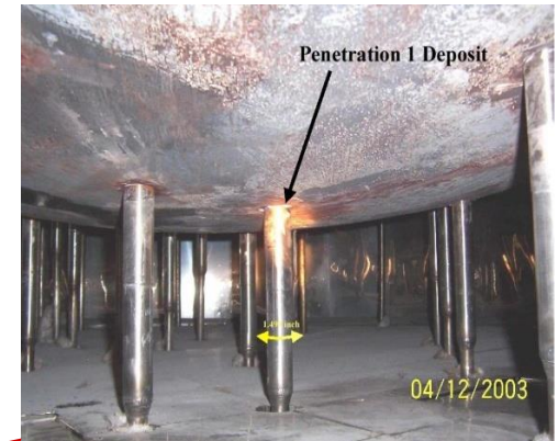
South Texas NPP, Reactor bottom penetration
